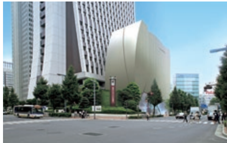
The new museum will open in May 2020 Photo image provided by Taisei Corporation First-Class Architect Office
